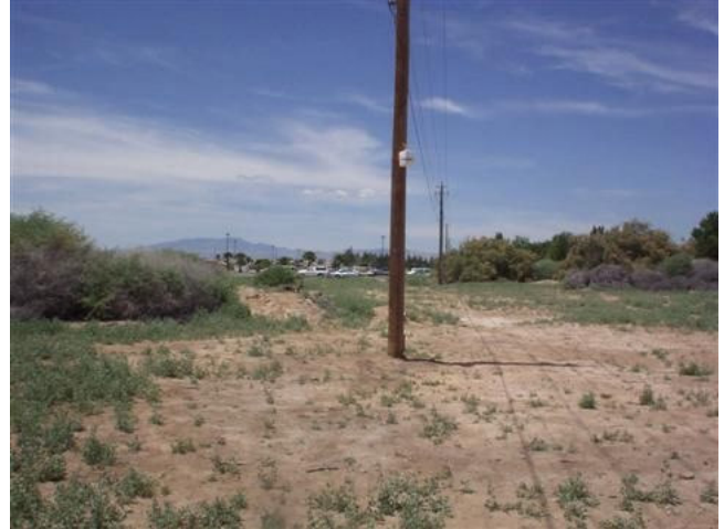
Figure 3-3. Sampler Mounting on a Utility Pole
